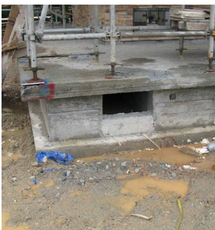
(a) During construction
