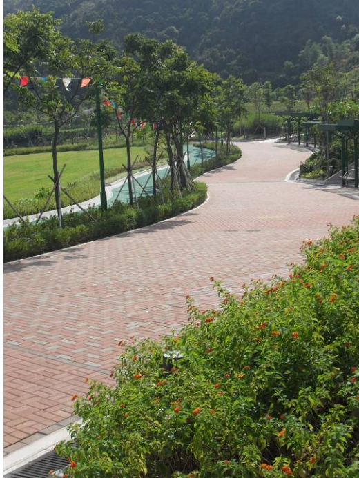
Photo 8 Pavement with concrete blocks
