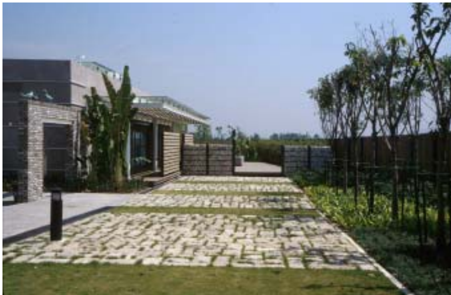
Figure 1 Southern entrance of Phase 1 building with recycled granite as paving
