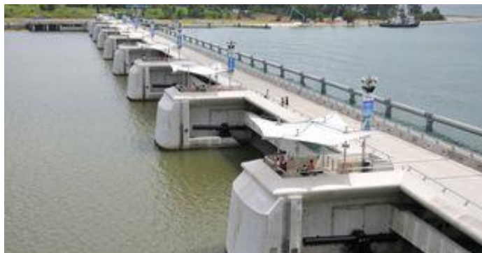
Figure 2 Overview of Marina Barrage [9]
