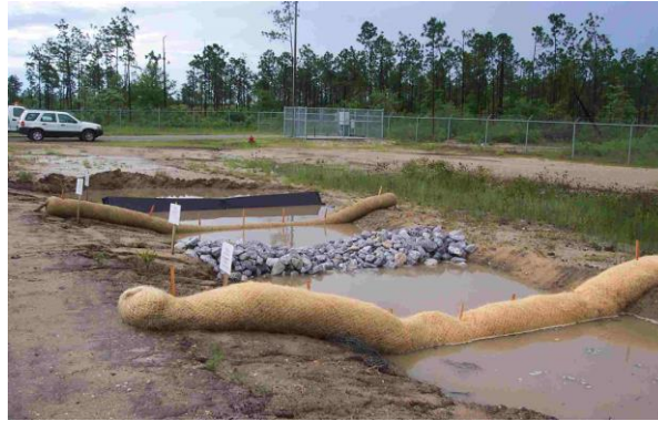
Figure 5 Sand and Organic Filter
