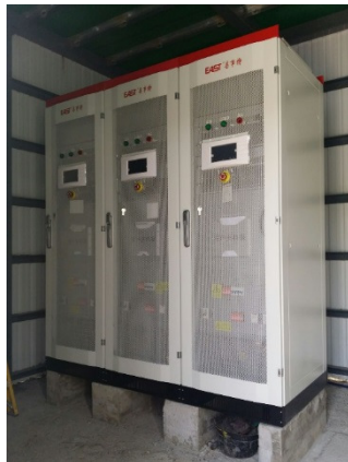
Fig. 11 DC-AC Inverters
