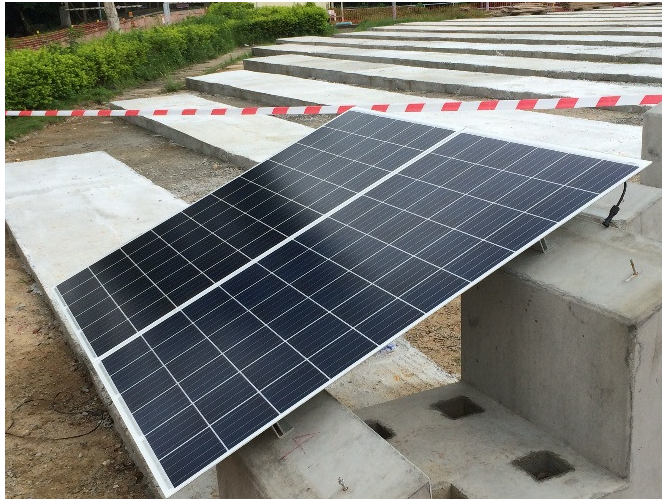
Fig. 5 Concrete Support for PV Panels
