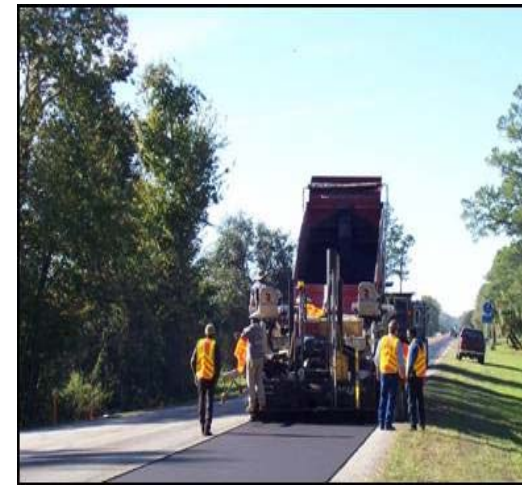
Asphalt Laying
