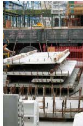
Semi-precast Slabs
