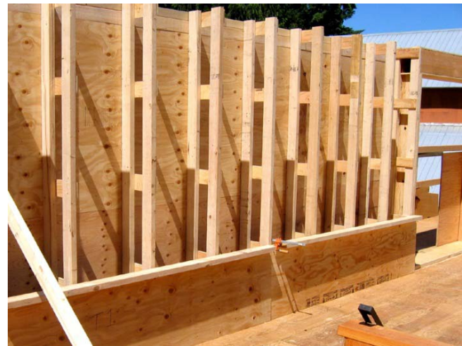
Timber Formwork
