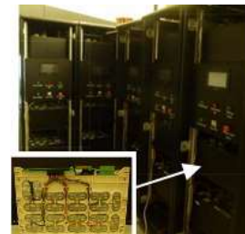
30 kVA Distributed Storage System
