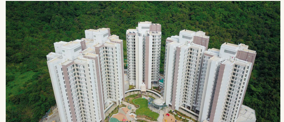
FSD's Pak Shing Kok Married Quarters in Tseung Kwan O, the first high-rise concrete MiC building in Hong Kong
