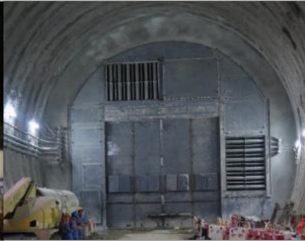
LTH BCP South Portal Northbound Tunnel Door, 2015, IL=37dB(A) (External view)
