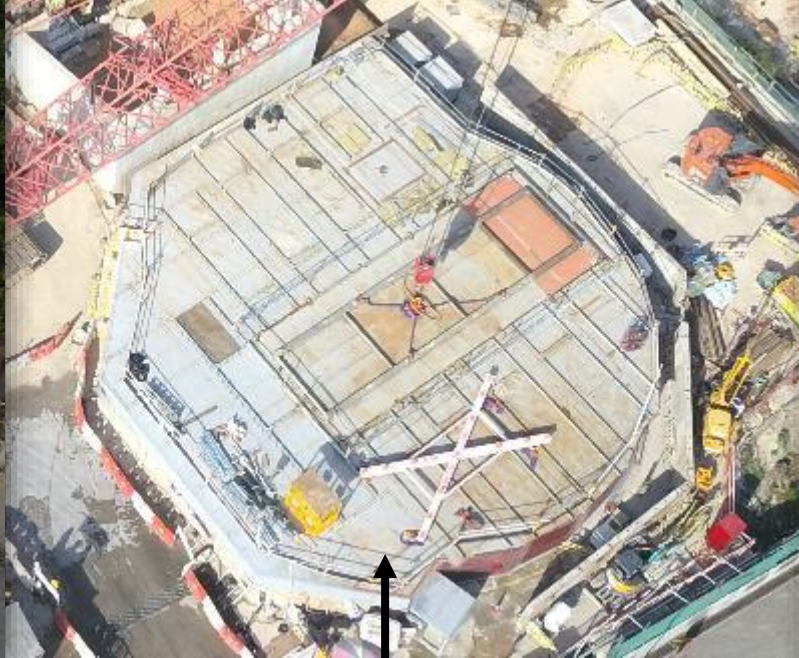
CKR HMT Shaft Enclosure, 2 nd Stage in 2019, IL=51dB(A) (Shape changed and removable cover enlarged to fit the construction need)
