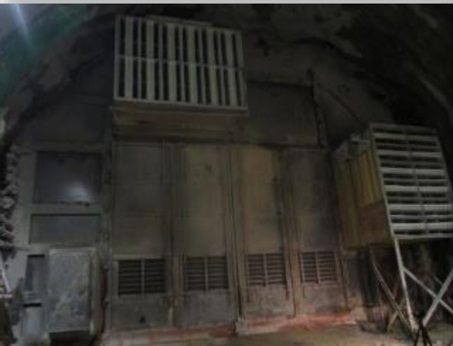
LTH BCP South Portal Southbound Tunnel Door, 1 st stage in 2015, IL=31dB(A) (internal view)
