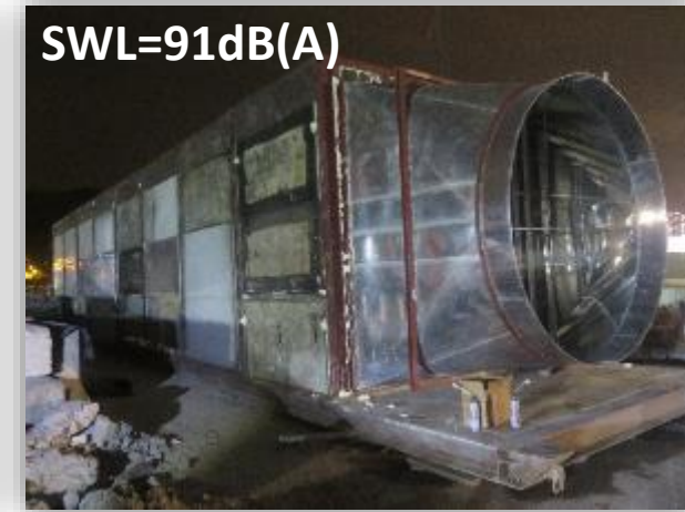
LTH BCP Enclosed Vent. Fans at Three Tunnel Portals, SWL=84-91dB(A) vs. 108dB(A) for standard one
