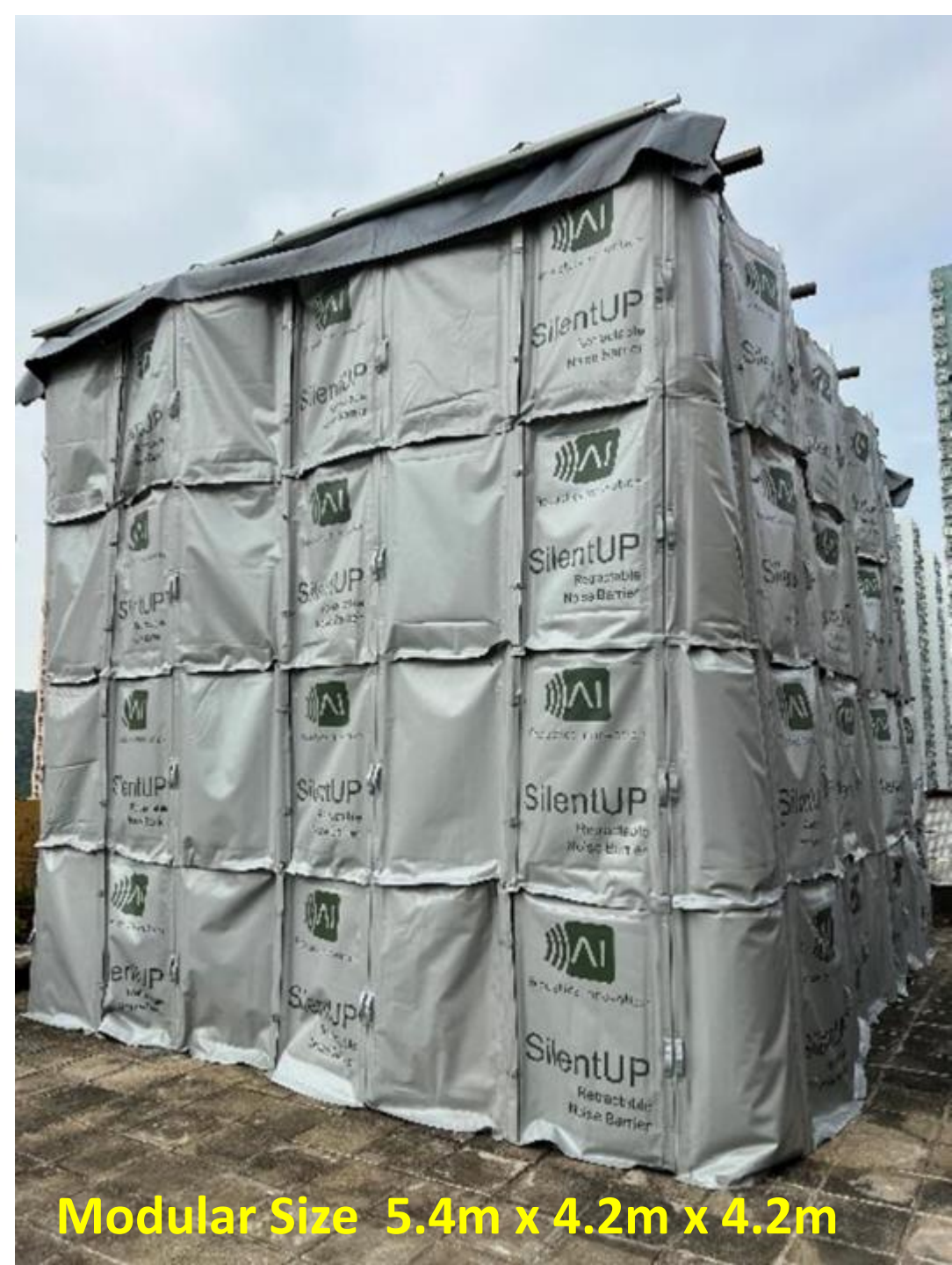
22m x 4.2m x 4.2m Long Enclosure by Modular Connections HKSAR ITC funded project
