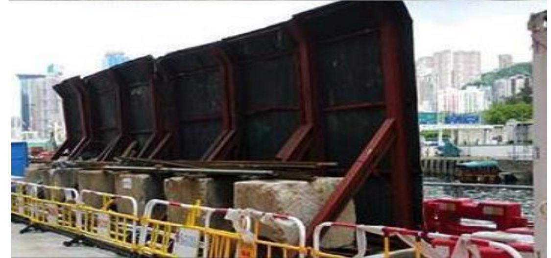
Movable Noise Barrier with concrete counterweight (max. ~3m high , movement by crane)
