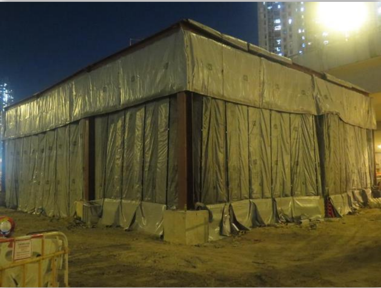
D-wall Construction Enclosure , 15x18x7m (H), 2020, IL=21-25dB(A) for white noise
