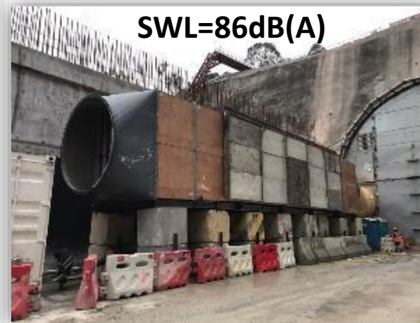
LTH BCP Enclosed Vent. Fans at Three Tunnel Portals, SWL=84-91dB(A) vs. 108dB(A) for standard one
