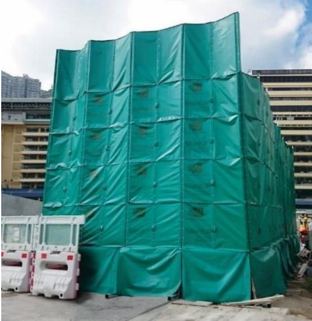
Retractable Noise Barrier (Erection without machine) Up to 7m high, on water barrier
