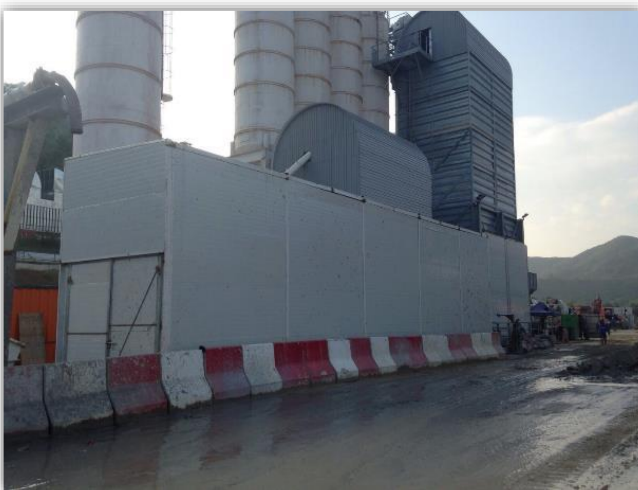
LTH BCP North Portal Enclosed Mortar Plant, SWL of Components=78-95dB(A)
