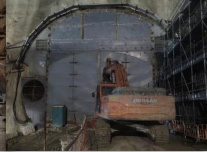
LTH BCP North Portal Northbound Tunnel Door, 2 nd Stage in 2016, IL=37dB(A)
