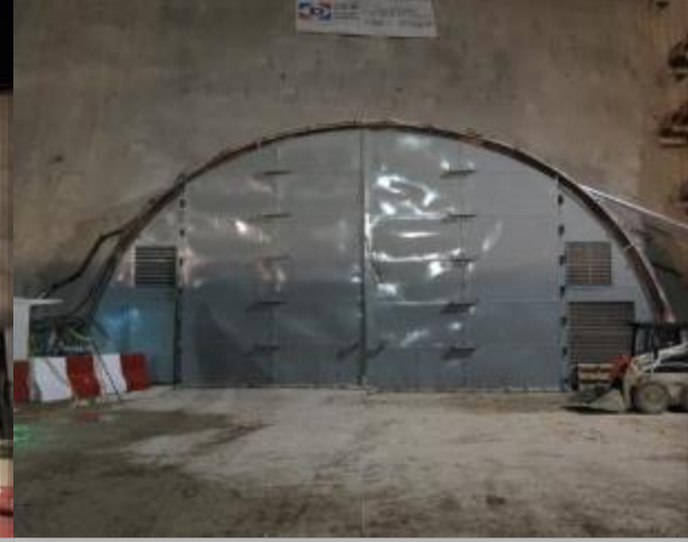
LTH BCP North Portal Northbound Tunnel Door, 1 st Stage in 2015, IL=37dB(A)
