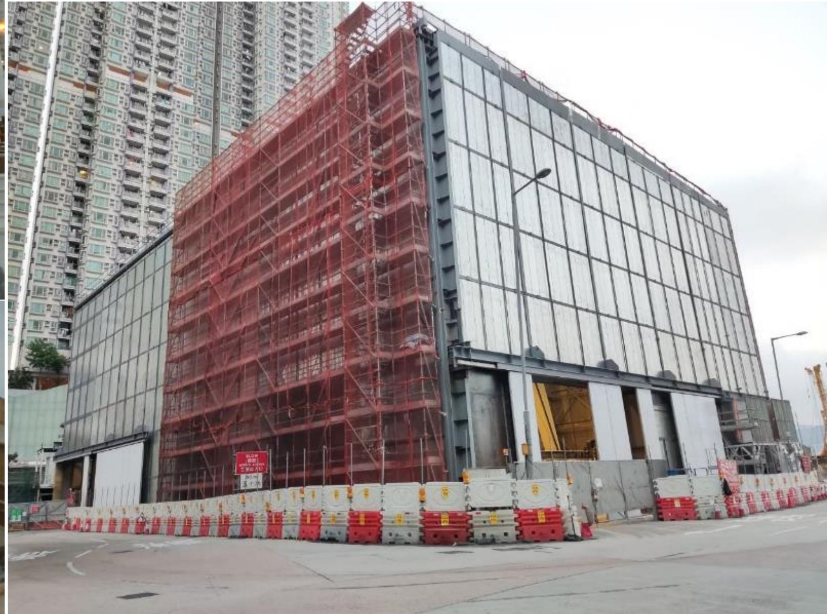
CKR MTK Enclosure, 2 nd Stage in 2021, IL=36dB(A)
