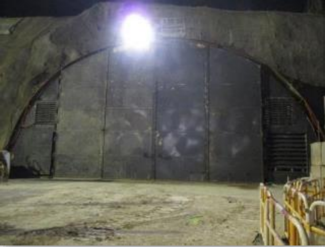
LTH BCP North Portal Southbound Tunnel Door, 1 st Stage in 2014, IL=42dB(A)
