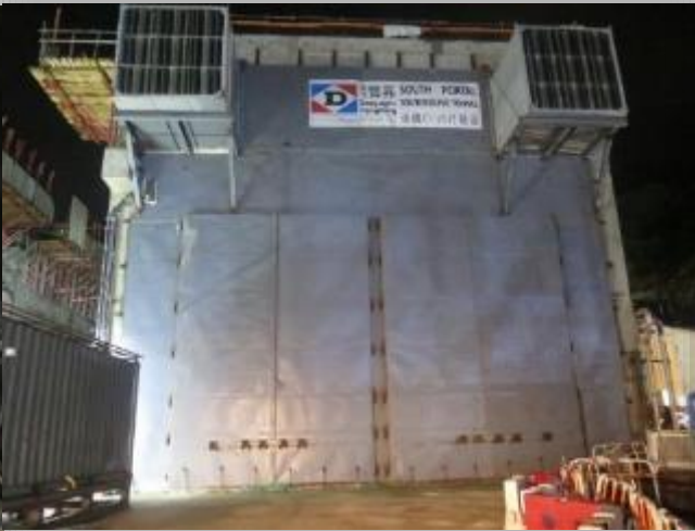
LTH BCP South Portal Southbound Tunnel Door, 2 nd stage in 2016, IL=34dB(A) (IL of left door=34dB(A), IL of right door=37dB(A))
