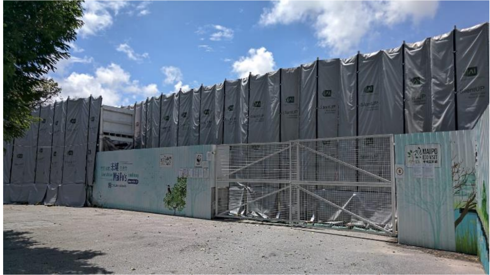
5m(H) x 105.3m(W) for 3 sides of the site boundary 4m (H) & 6m(H) x 45m(W) along 1 side
