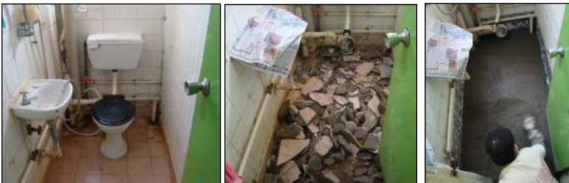
Figure 17: Time Consuming and Disturbing Conventional Re-waterproofing
