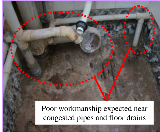
Figure 18: Problematic Areas for Conventional Waterproofing System
