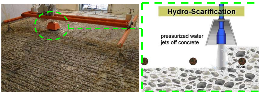
Figure 16: Concrete Removal by Automatic Hydro-Scarification Machine
