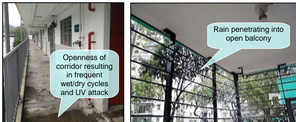
Figure 2: Exposed Elements in Aged Public Housing
