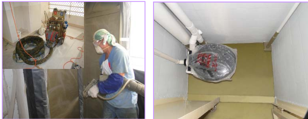
Figure 19: Spray-on PWS to Cope with Congested Areas
