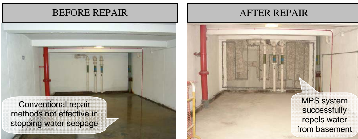
Figure 12: Basement Conditions before and after the Installation of the MPS system
