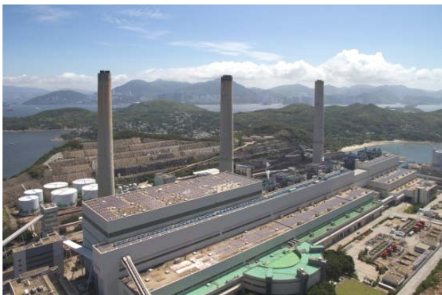
Fig. 2 – TFPV in Lamma Power Station
