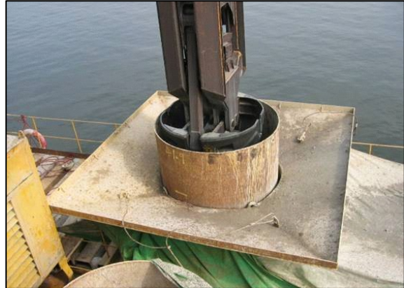
Figure 12 – Y-Shaped Funnel over Piling Case
