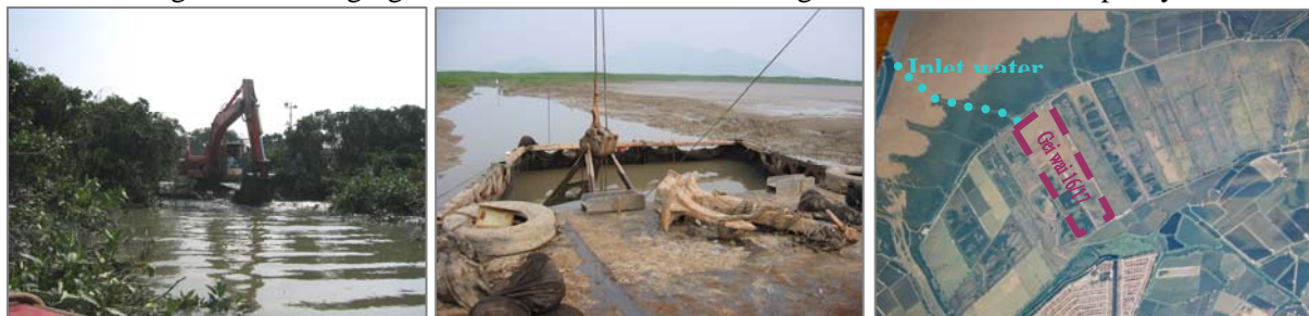
Figure 6 – Dredging of Inlet Water Channel Linking Gei Wai 16/17 to Deep Bay
