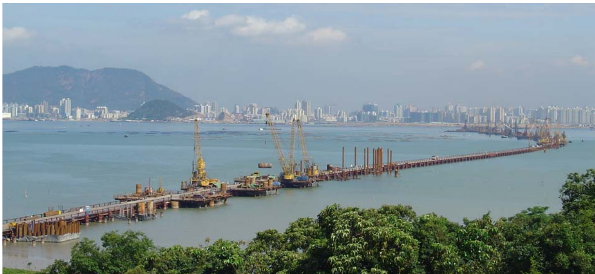
Figure 10 – Temporary Access Bridge (TAB)
