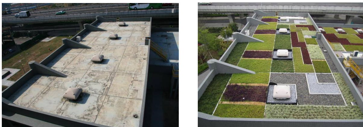
Figure 1 : Before and After Retrofitting of Green Roof at Sha Tin Sewage Treatment Works
