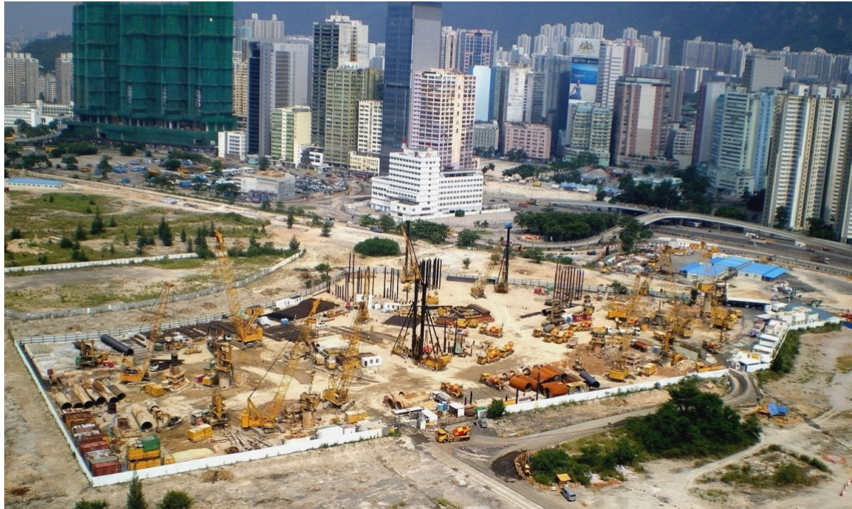
Figure 2 – Bird's Eye View of Kai Tak Development Site 1A at piling stage
