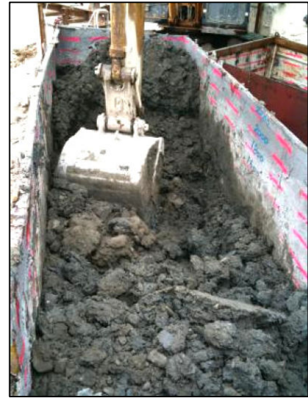
Figure 10 - Mixing of Ingredients with a Backhoe
