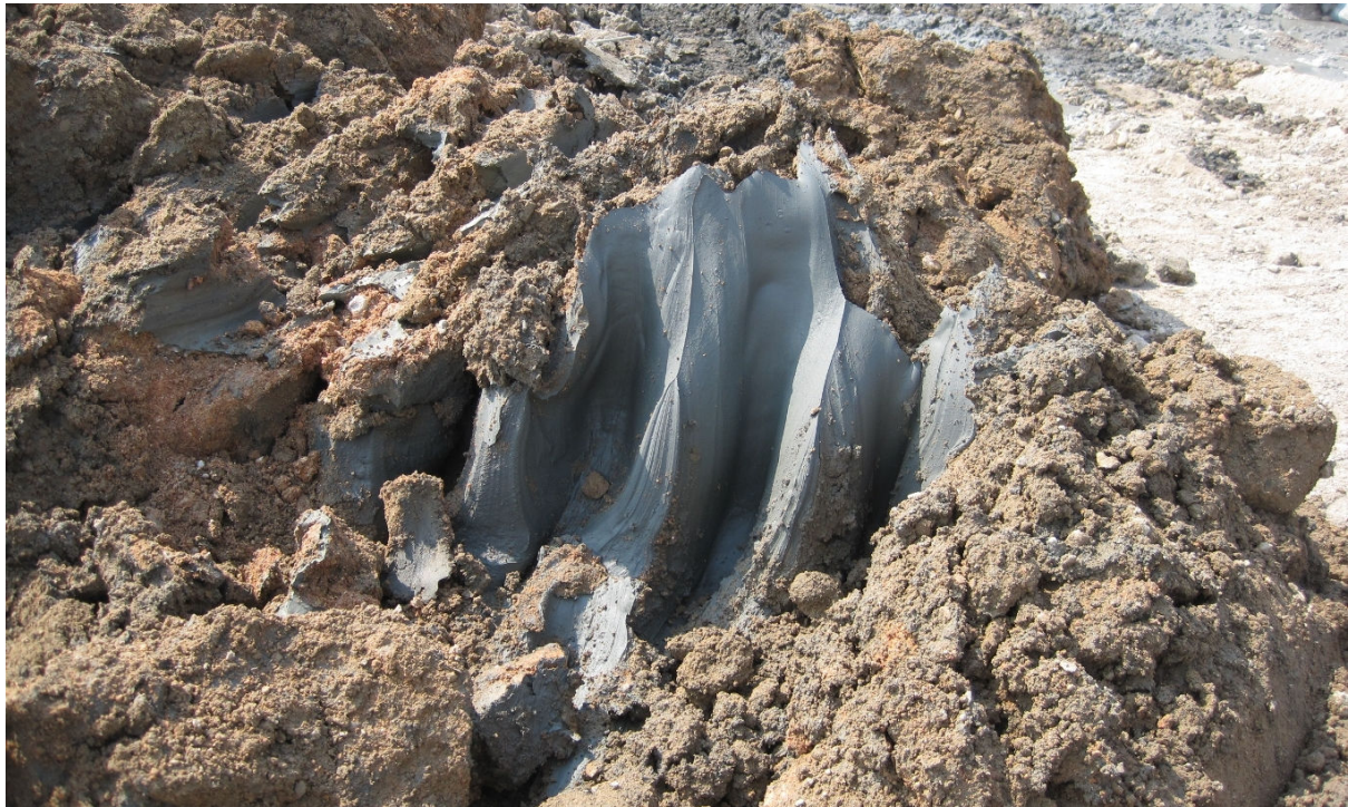
Figure 4 – Marine mud being excavated
