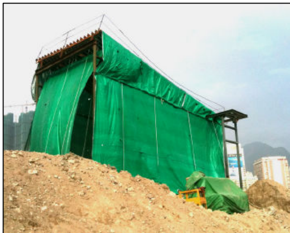
Figure 12 – Temporary Dust Screens
