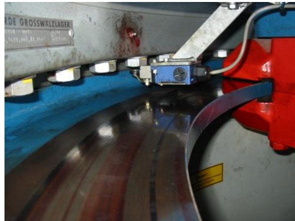
Fig. 9 Rust particles accumulated on the yaw brake-disc may generate high pitch noise.
