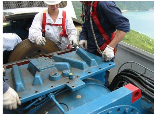
Fig. 5 Routine Maintenance of Wind Turbine
