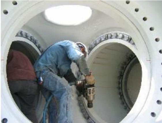
Fig. 6 Adjustment of the pitch angle to the required value by loosening and re-tightening the bolt.
